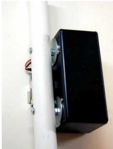
Box mounted with 10-32 X 1/2" Screws & Fender Washers
